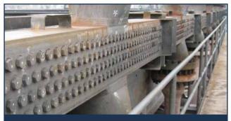
The Curran method eliminates containment setup on catwalks, thus keeping headers unencumbered and accessible.
