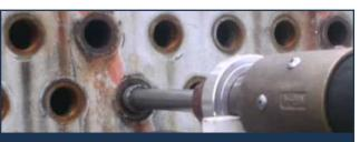
Curran specialized nozzles "bridge" and capture waste-grit and tube debris tube-end to tube-end.
